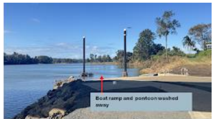
Figure 11. From L-R, (L) the boat ramp and pontoon in situ at the Rocks Ferry reserve prior to the 2025 flood, and (R), the pontoon and ramp washed away
