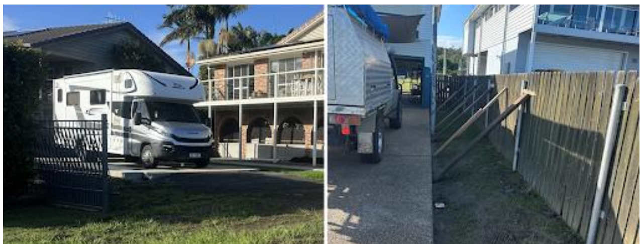
Figure 8. Experience with flooding in 2021, these residents on Settlement Point Drive in Port Macquarie have increased their own personal resilience by making preparations to protect personal property. (Image on left) – shows a newly constructed elevated concrete slab and new motorhome which avoided inundation on this occasion. (Image on right) – after losing fences in 2021, this resident has reinforced fences with temporary timber bracing and galvanised steel poles with concrete footings (Image taken facing away from river)
