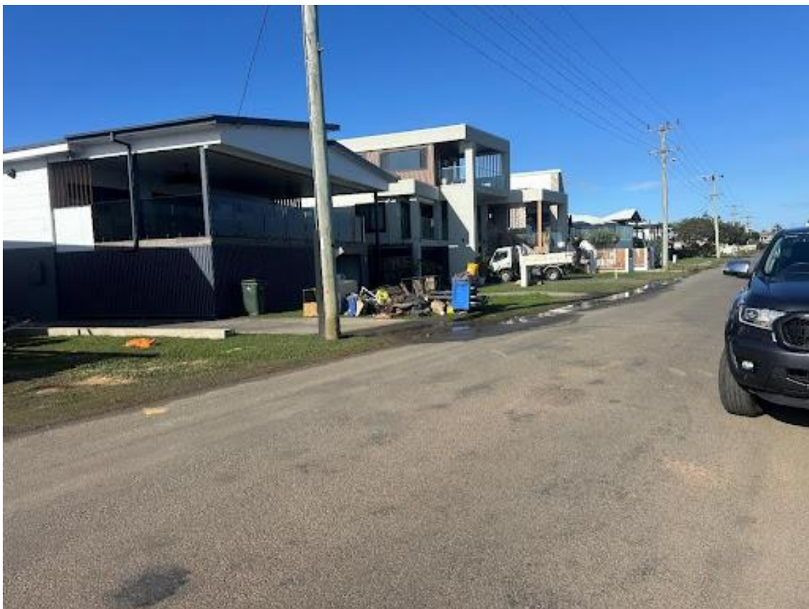
Figure 9. One of only several houses on Settlement Point Drive Port Macquarie with flood insurance costing ~ $5000 per year. Most houses on the street are raised on piers with living areas located on first floor and ground floor is largely a concrete shell / garage / storage which allows for waters to pass through
