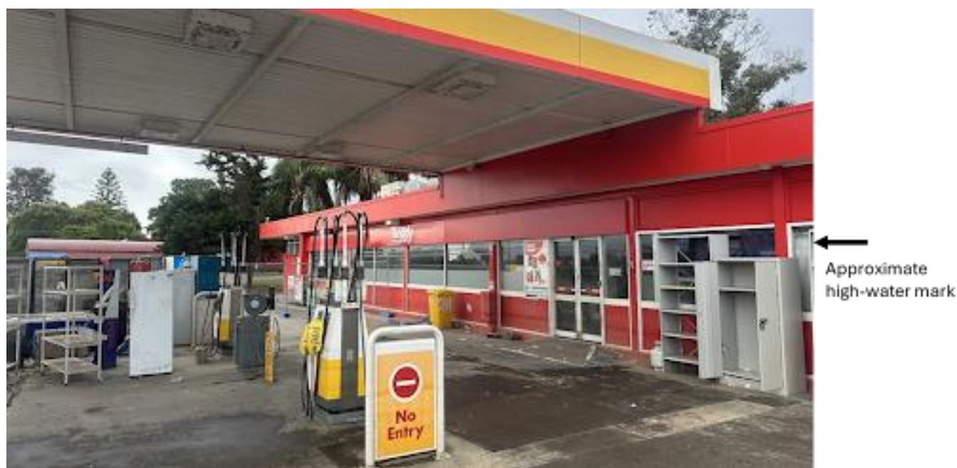
Figure 4. A service station in West Kempsey remains closed with the remnants of fuel bowsers, fridges and freezers destroyed in the flood behind tape. Flood level at this location was > 2 metre
