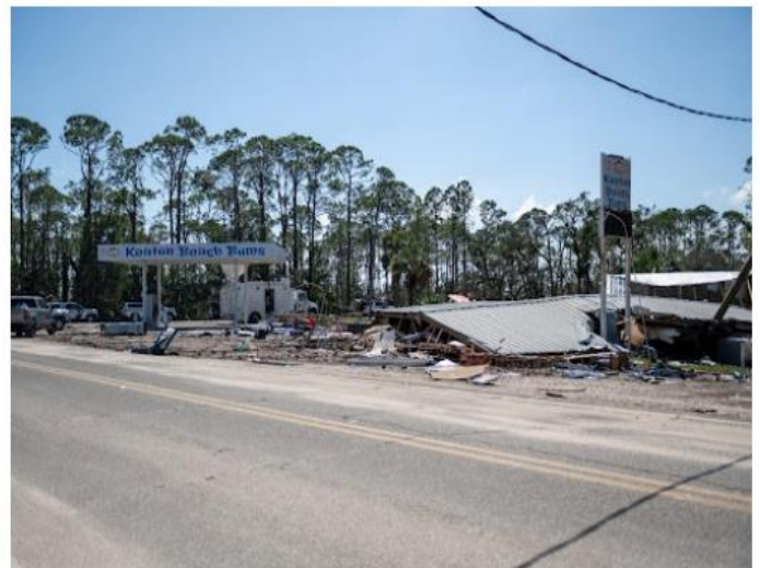
Figure 4. Buildings flattened from Helene's storm surge in Keaton Beach, Florida, United States. Source: USCG South East.
