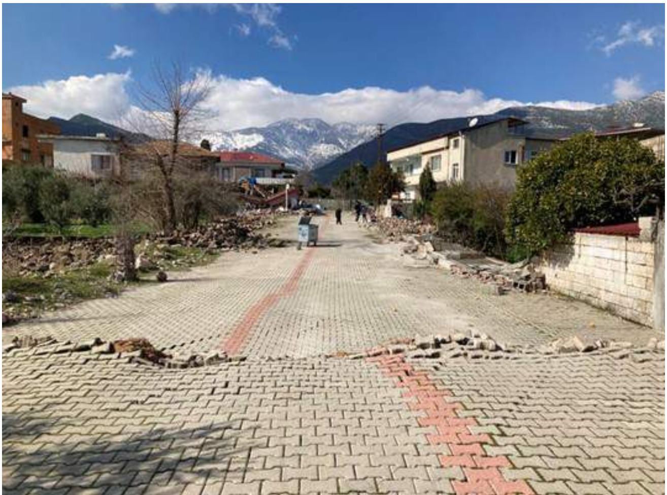
Figure 8. Offset railway in Narlı (located near Pazarcık, southeast of Kahramanmaraş in Figure 2). Fault strands appear to run across the railway in the near and middle distance, with left-lateral displacement. A strong ground motion recording in Pazarcık (near this railway) is shown in Figure 10. Source: H. Serdar Akyuz (2023).
