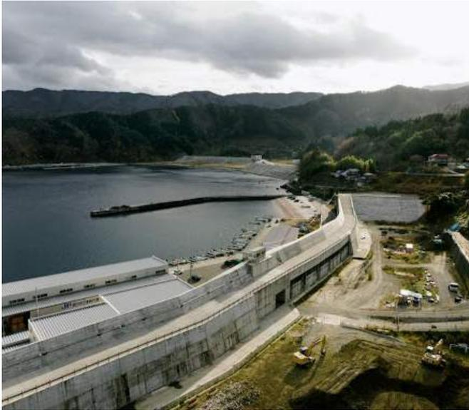
Figure 3. A new 14-metre-high seawall near Toni in the city of Kamaishi, Iwate Prefecture. The old seawall was 12 metres high but could not withstand the 2011 tsunami.
