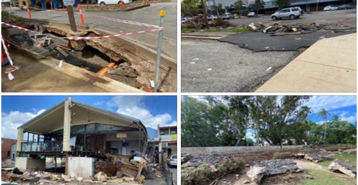
Figure 5: Examples of structural damage in the Lismore CBD. Clockwise from top left - stormwater drain and gutter, car park surface, a stone wall adjacent to the Richmond River and the rear bar of the Richmond Hotel.
