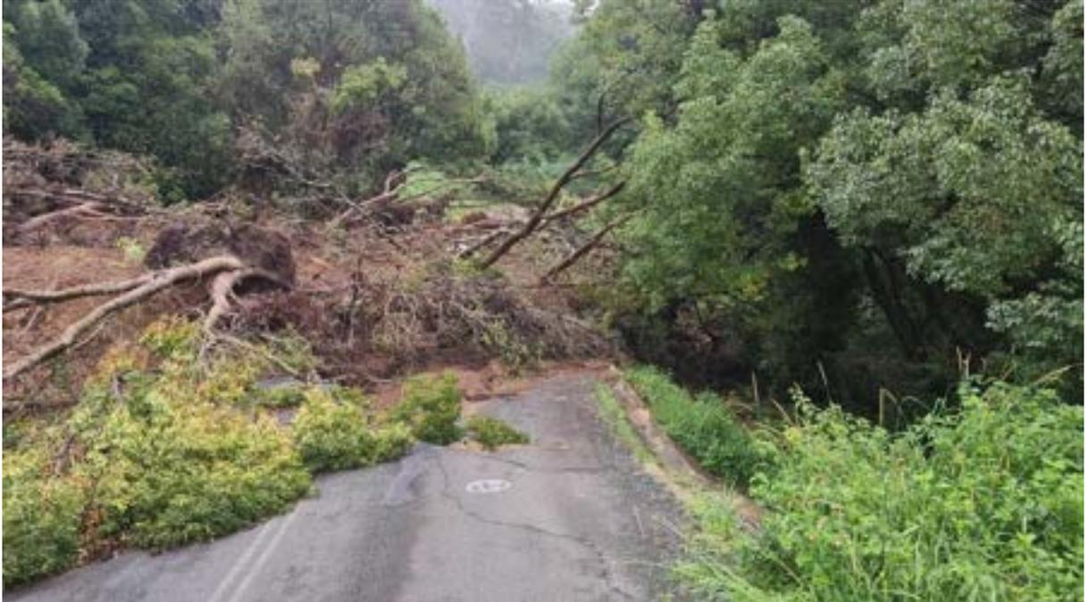
Figure 16: A landslide in the Wilsons Creek catchment, south of Main Arm, completely blocking a road near Federal (Image source: Local resident known to survey team).
