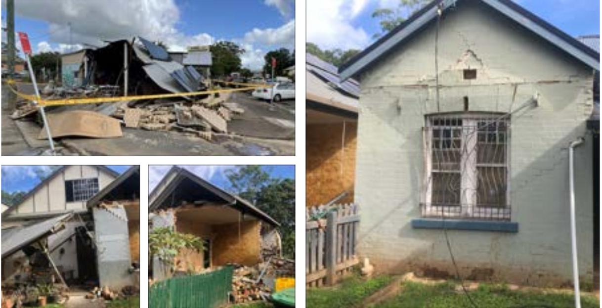
Figure 7: Examples of structural building damage in South Lismore
