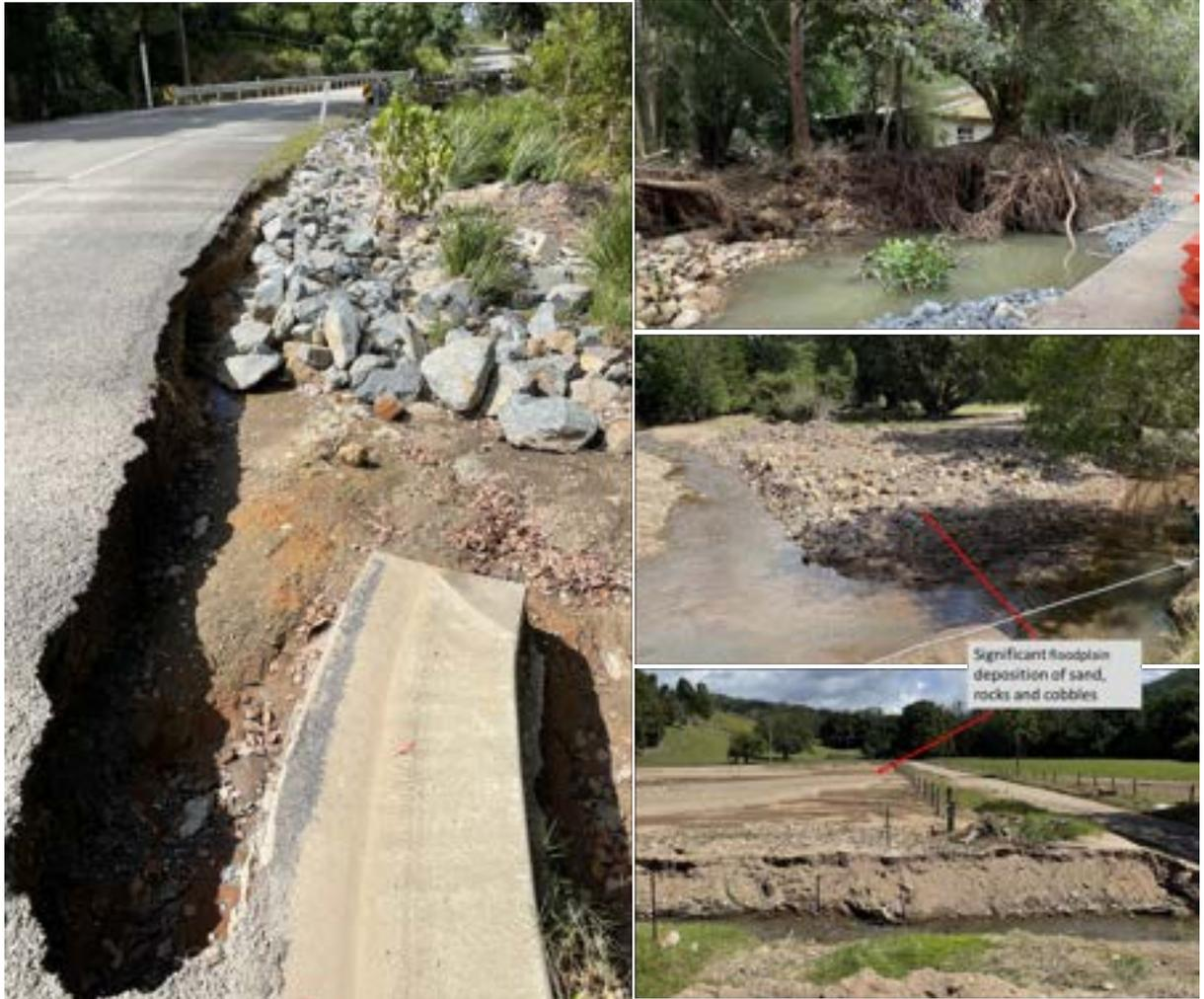
Figure 17: Road base and soil erosion from roadways and tree roots (left & top right) and evidence of fluvial geomorphic change with the deposition of sand, rocks and cobbles on floodplains (mid and bottom right) caused by deep and fast flowing flood waters in the confined Brunswick River catchment between Main Arm and Upper Main Arm.
