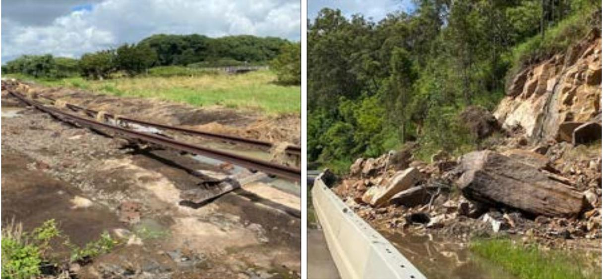
Figure 4: Washed out railway line (left) on Naughton Road between Casino and Lismore and a rockslide (right) closing one lane of Bentleys Road approximately 10km from South Lismore.
