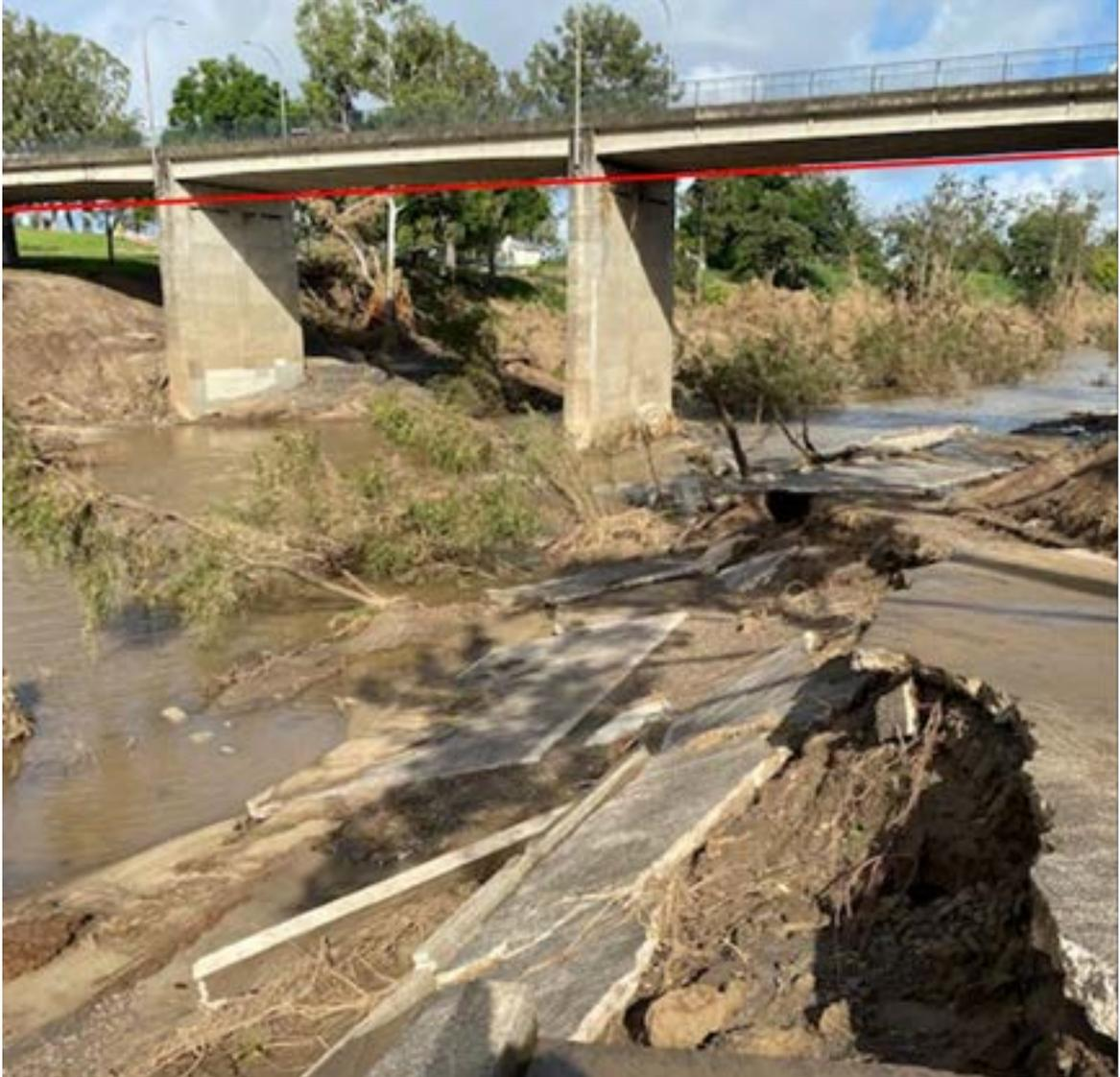
Figure 3: The Richmond River in Casino beneath the Irving Bridge. Red line indicates the approximate peak height of flooding on the 27th of February. Note the destroyed roadway and trees lain over by the force of flood water.
