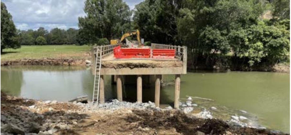
Figure 15: The bridge on Main Arm Road between Mullumbimby and Main Arm, showing a large section washed away by the Brunswick River two weeks earlier.
