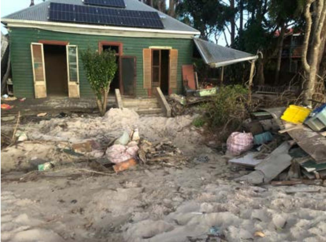
Figure 10: Broadwater residence showing structural damage and large amounts of flood-deposited sand in the front yard.
