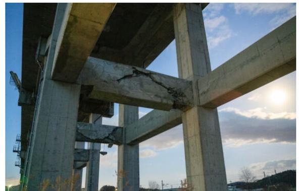
**Figure 3:** Left: derailed bullet train on bridge near Shiroshi, Miyagi Prefecture. Source: Mainichi Shimbun. Right: Damaged bullet train viaduct Source: Xinhua/Zhang Xiaoyu.
