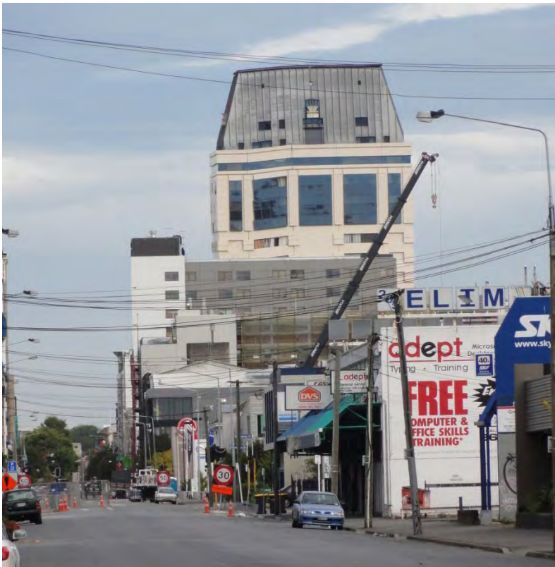
Figure 8. The noticeable lean and kink of the Grand Chancellor Hotel.
