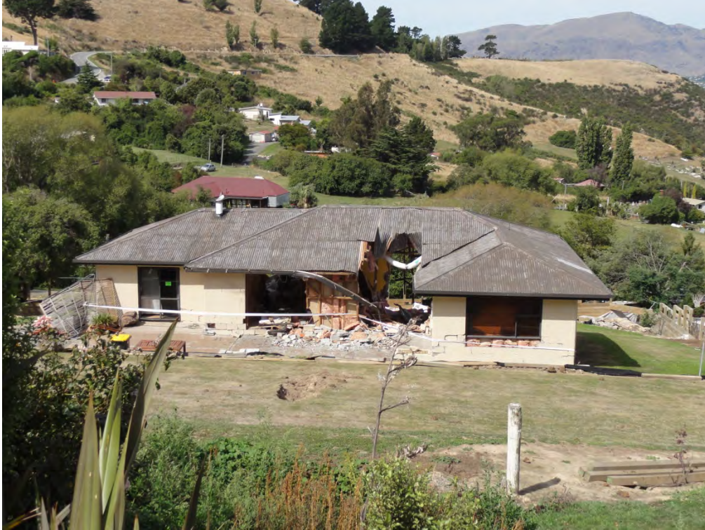
Figure 5. Damage to home due to falling boulder.
