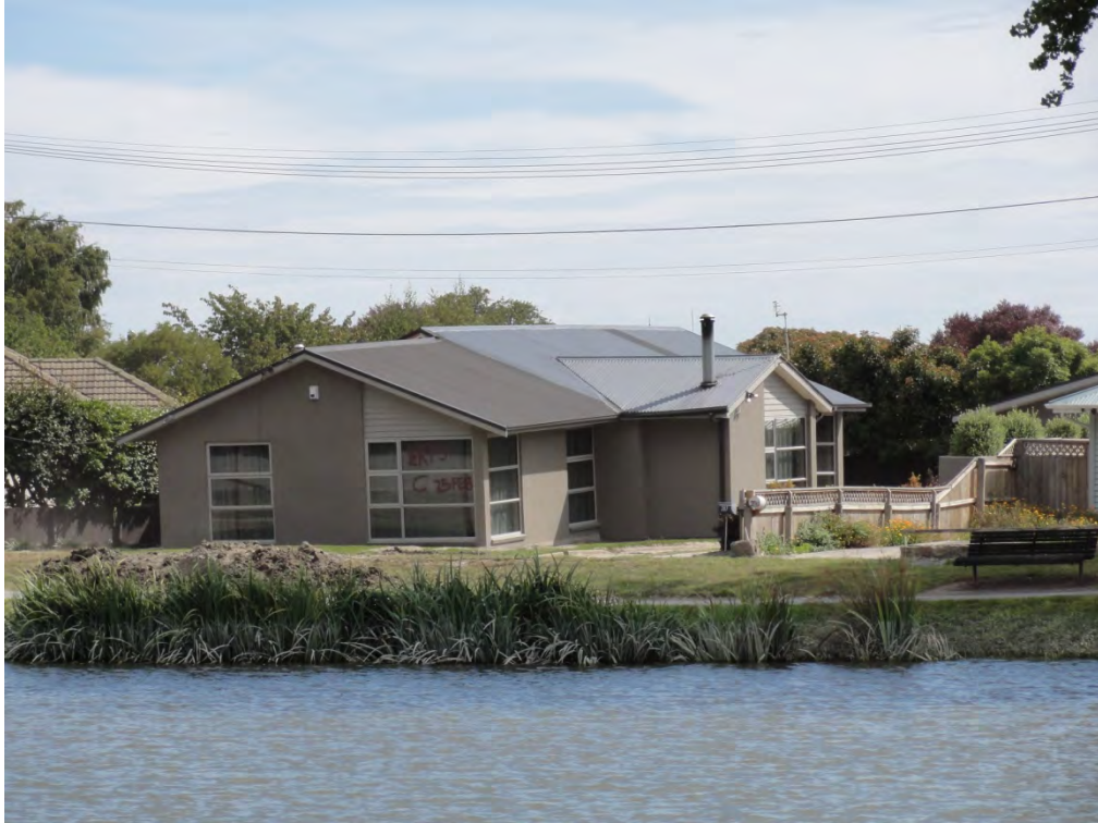
Figure 5. Tilting of home most likely due to lateral spreading.
