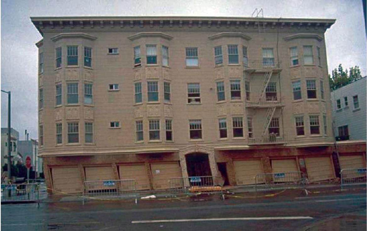
**Figure 3.** Building damaged in San Francisco in the 1989 Loma Prieta earthquake. Source: Raymond B. Seed.
