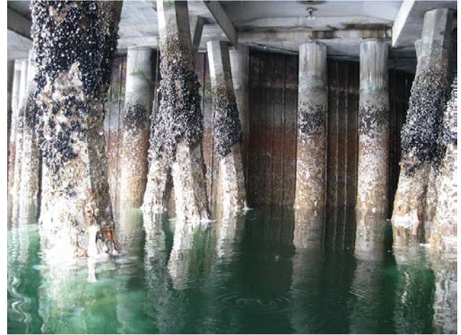
Figure 1: Erosion due to sea water on concrete pylons. Image: Brian Robinson.
