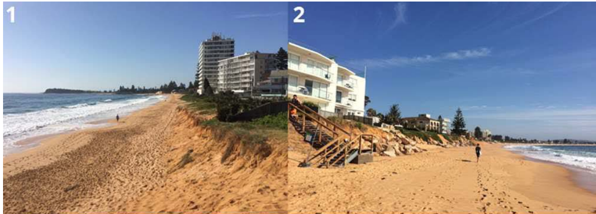
Figure 3. Beach and dune erosion at the south end of Collaroy-Narrabeen beach in Sydney, caused by a clockwise rotation of the shoreline under southerly wave conditions (photographs taken by Andy Short, 2015). Beach width (foot of dune to water line) can vary on the order of 15 - 20 m during rotation episodes.
