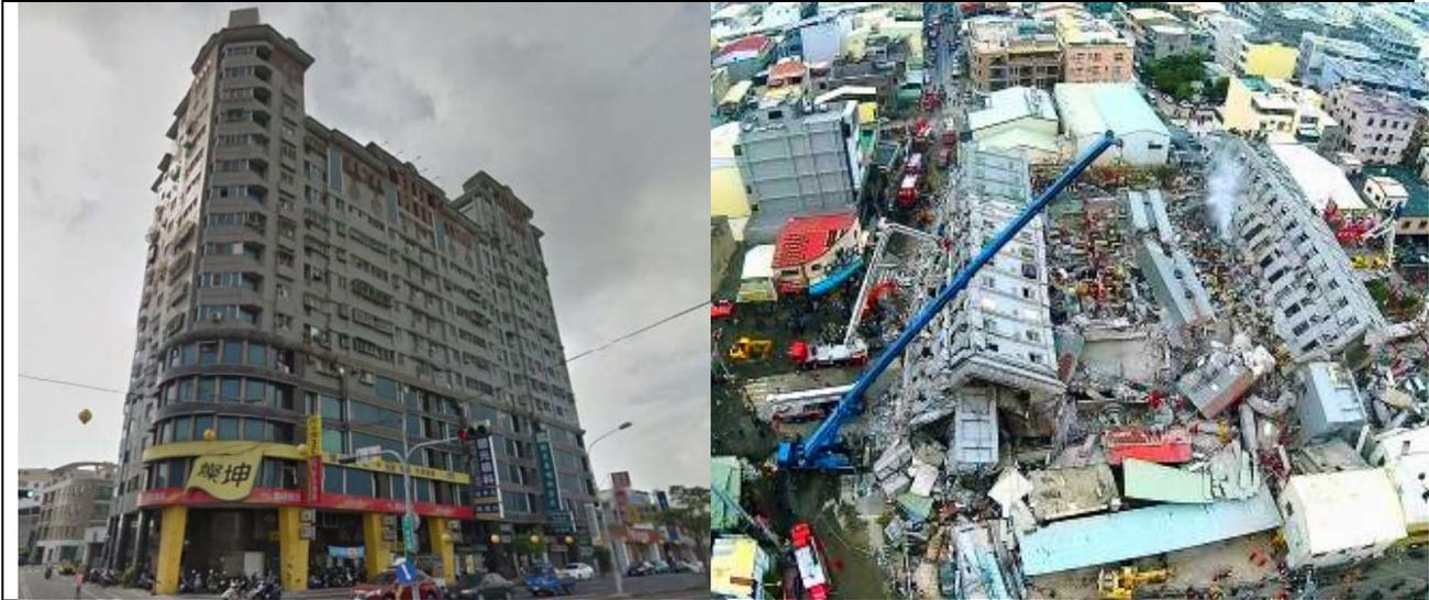
**Figure 3.** The Weiguan Jinlong residential building in Tainan before (left) and after (right) collapse. The surrounding buildings do not appear to have severe damage (Photo: Taipei Times).
