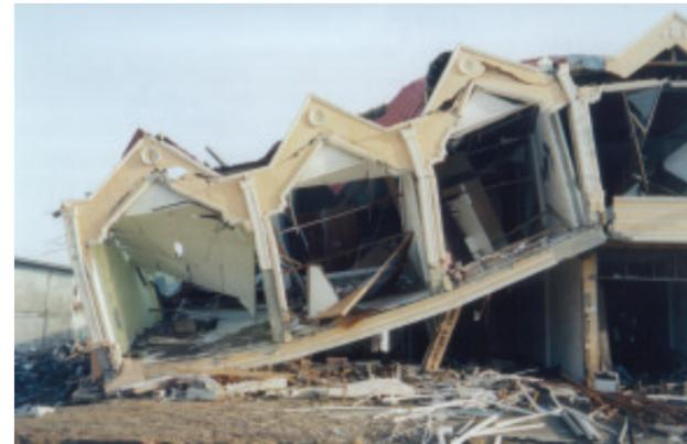
**Figure 5:** A building with a structural wall taken out by the force of water or floating debris.
